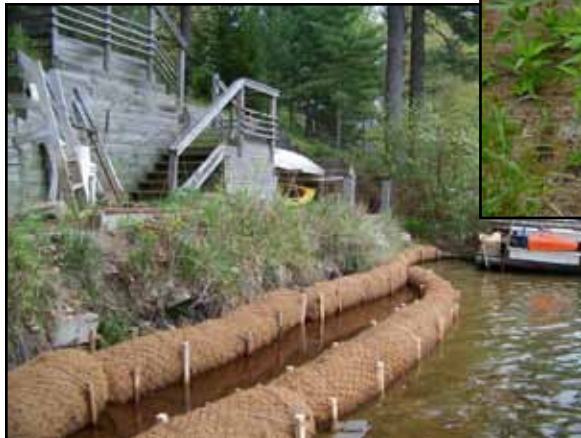
A newly-installed shoreline erosion-control project.
